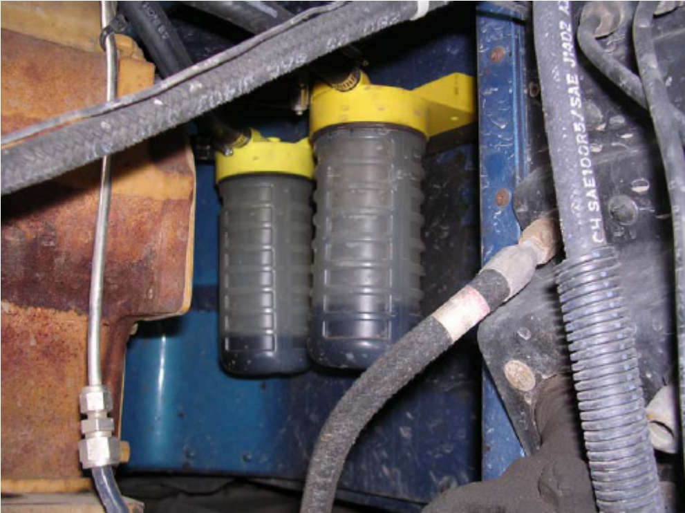
Figure 5: New Condensator CEAS system installed on the test vehicles firewall.
